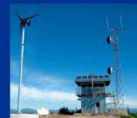
Telecom stations power
